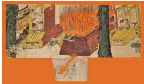
"Kakesumiya Iron Mine," from the private collection of Masahiro Kake, detailing production methods used in traditional Japanese iron mines.
